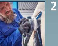
For the next step, use a orbit sander, sandpaper or sanding pad to dry grind the surface. Clean the area again with a recommended cleaner, as the **DINITROL 7660**, to ensure that the substrate is free from dust and substances that disturb the lacquer wettings. If the car has been ground down to the metal, the affected surface needs to primed.
