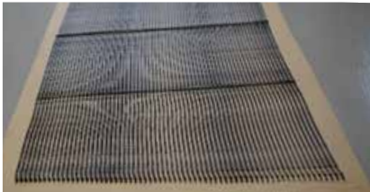
Fig. 2: Adhesive application using adhesive comb
