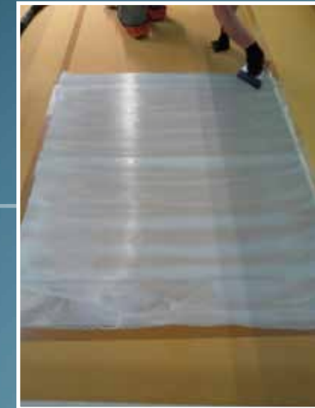
Fig. 9: Even distribution of the adhesive with a trowel
