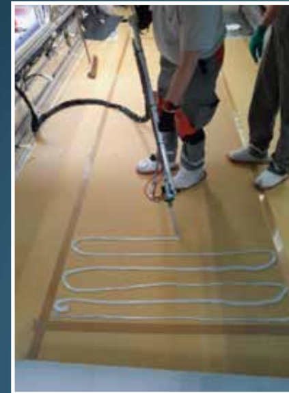
Fig. 7: Adhesive is distributed with the machine
