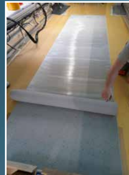
Fig. 8: The floor covering is carefully laid and rolled on
